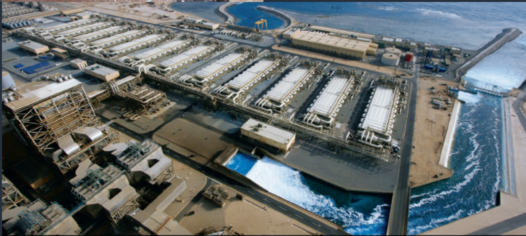
Doosan Heavy - Seawater desalination plants
